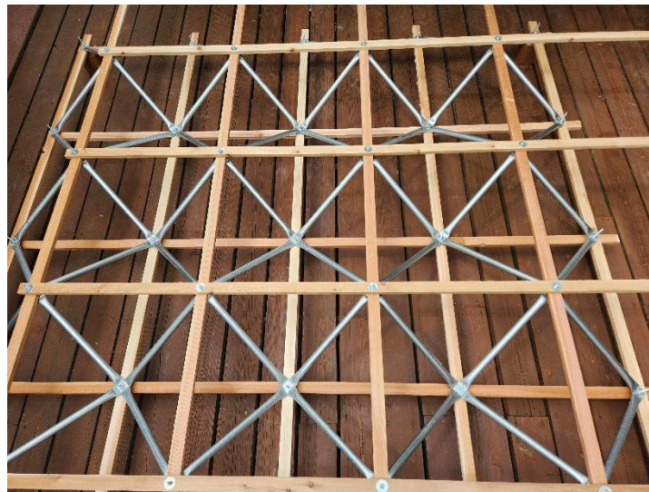
Figure 15b: Top-view of 8'x8' Wood-Steel spaceframe sub-section.
