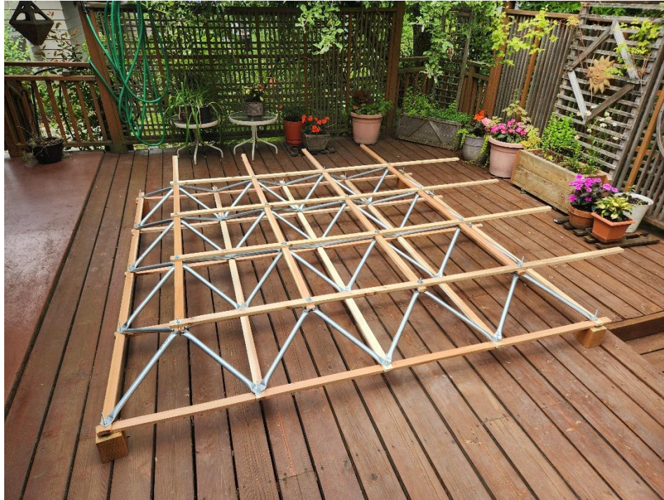
Figure 15a: Assembled 8'x8' Wood-Steel spaceframe sub-section.
