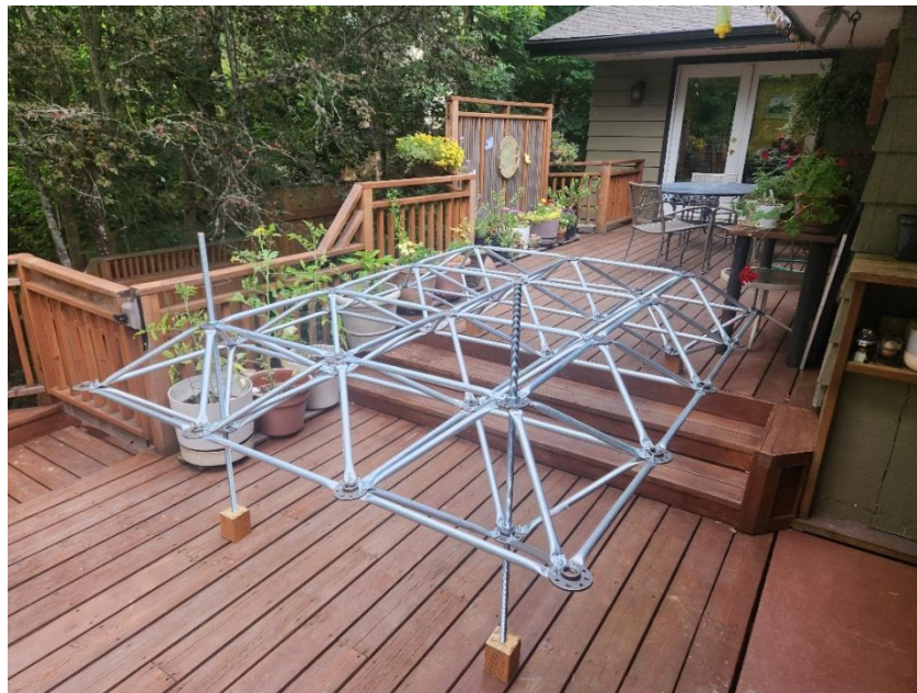
Figure 11: Spaceframe using the Ring Node with level adjustable corner posts.
