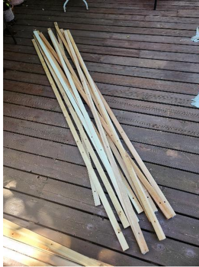
Figure 13: Wood boards with holes drilled. These will crisscross to make the square chords.
